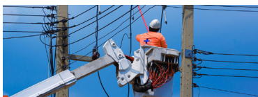
Pole & Transformer Inspections
